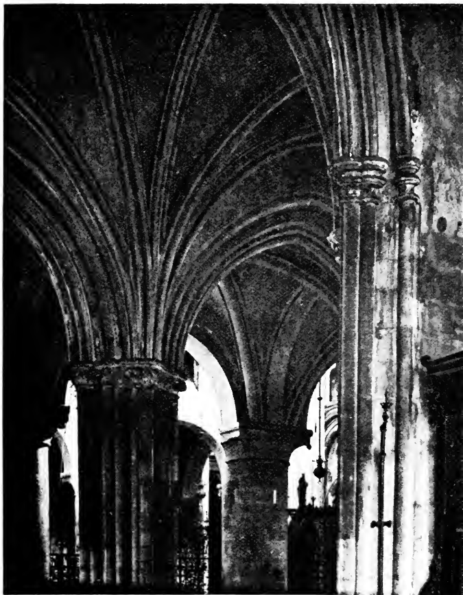
FIG. 36. VAULT-RIBS IN CATHEDRAL
